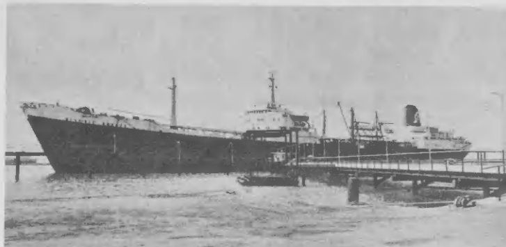
With the second phase of reconstruction work completed, the West Pier was placed back in service on December 24, 1971 as a safer and more permanent facility.
